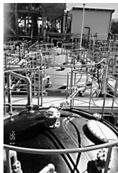
Level measurement in open reservoir with Two-Part System in a sewage treatment plant
