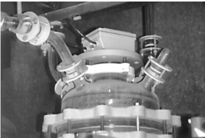
Measurement of various chemical ingredients with Compact Transmitter in a pharmaceutical plant
