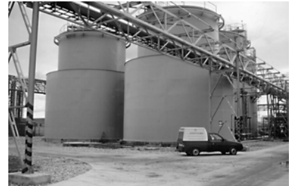
Measurement of 22 m high liquid fertiliser tanks with Compact Transmitters
